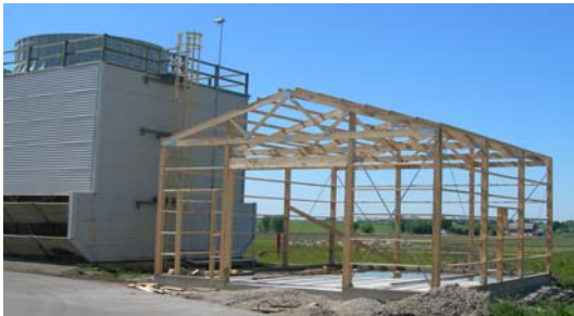
Chemical Storage Building
