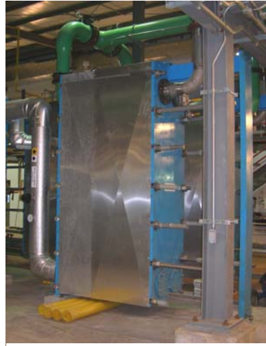
One of Four Completed Mash Cooler Expansions
