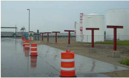
Construction of a Second Ethanol Truck Loadout Station Currently Underway
